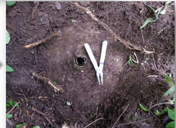
Excavation to Confirm Well Location
