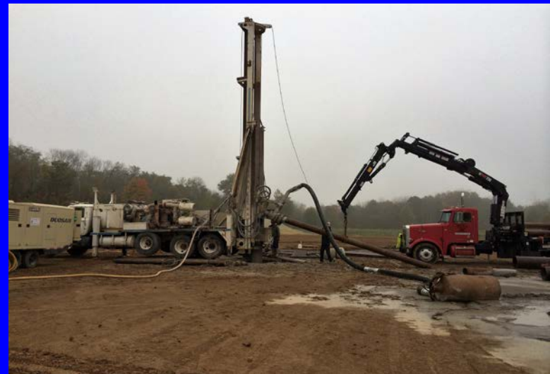
Concentric Casing Drilling Rig: inner drill pipe rotates an air percussion hammer/bit inside 94# 20" which is locked in place with a lock ring swivel and rotated independently of the inner drill pipe
